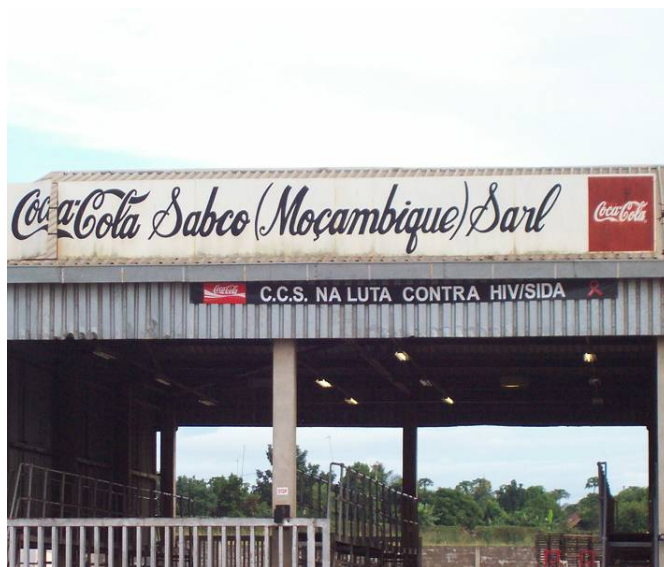
Photograph 3: Front View of Coca-Cola's Facilities in Nampula.
